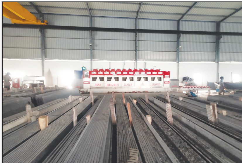
Granite Processing Unit financed by APSFC
